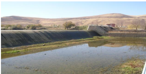
Figure 1. View of the Yusufkand Mahabad diversion dam and its ogee spillway
