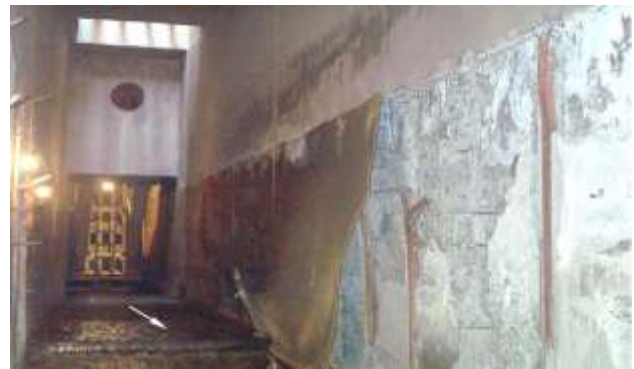
Figure 2. Damages in Sefidroud dam
