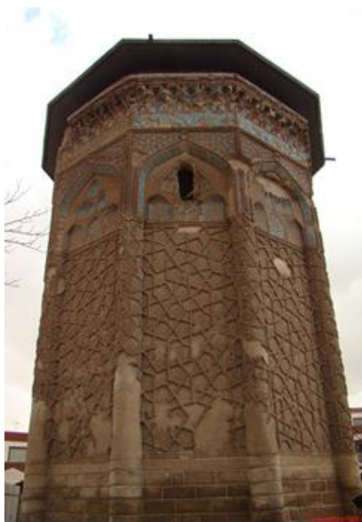
Figure1. General view of the Kabud Tower
