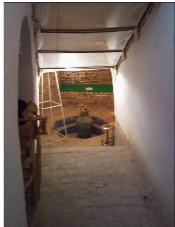
Figure 11: the path to direction air flow to the lowest part to shallow
