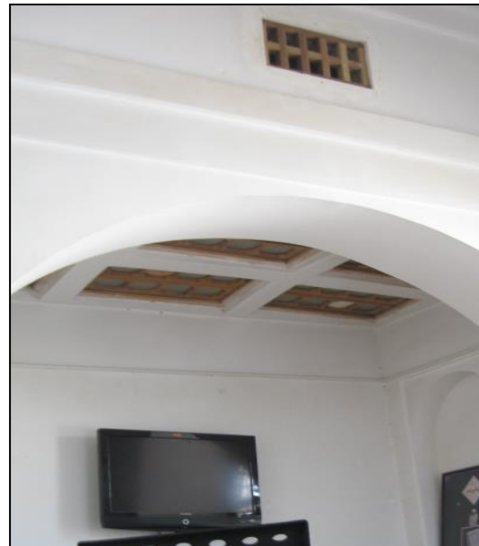
Figure 9: installed trap-door on the stem of the wind catcher and closing the lower trap-doors.
