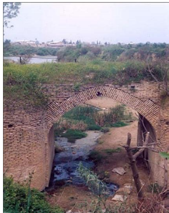
Figure 7. Today view of bridge
