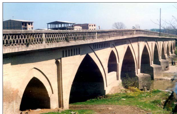
Figure 4. Today view of bridge
