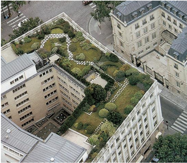
Figure 8. An Example of an Intensive Green Roof
