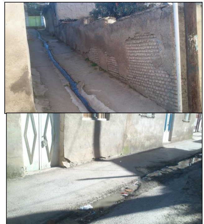
Figure 2. Bad condition of sewage system and dirt alley ways of Hassan neighbourhood of Gorgan (2013)
